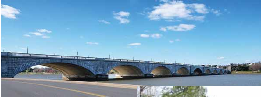
Arlington Memorial Bridge, DC/Virginia
